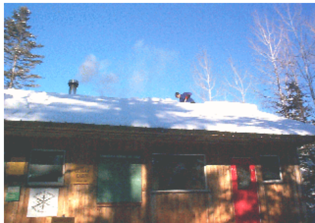
A volunteer shoveling snow off of the Cossar Cabin roof.
